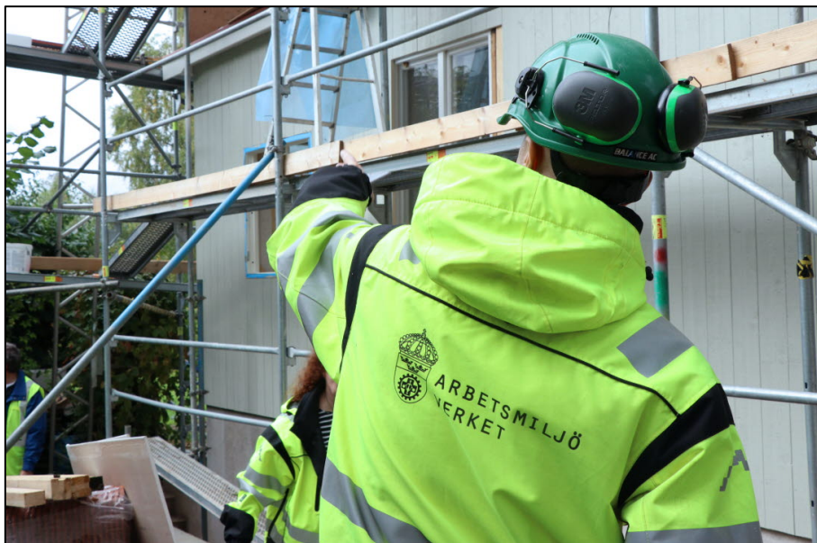
Photo 3. Inter-agency inspection of a construction site.
