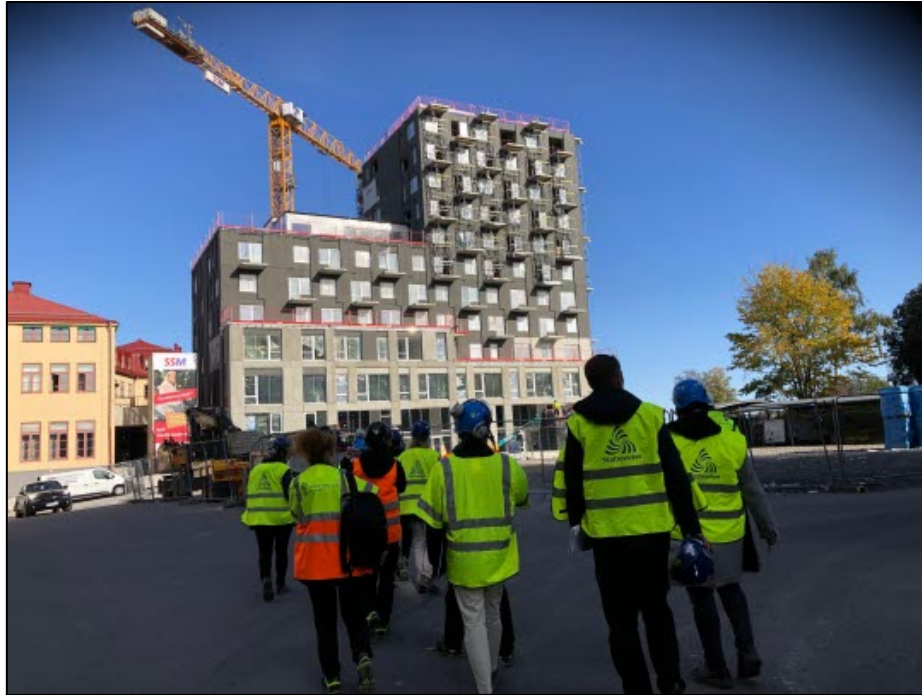
Photo 1. Inter-agency inspection of a construction site.
